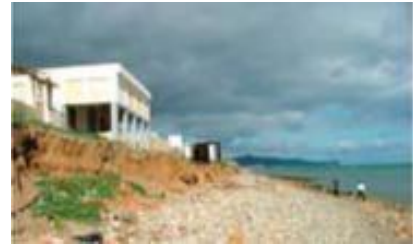
Erosion of Bouznika beach due to heavy swells in January and February 2014. Photo: 3rd national communication
